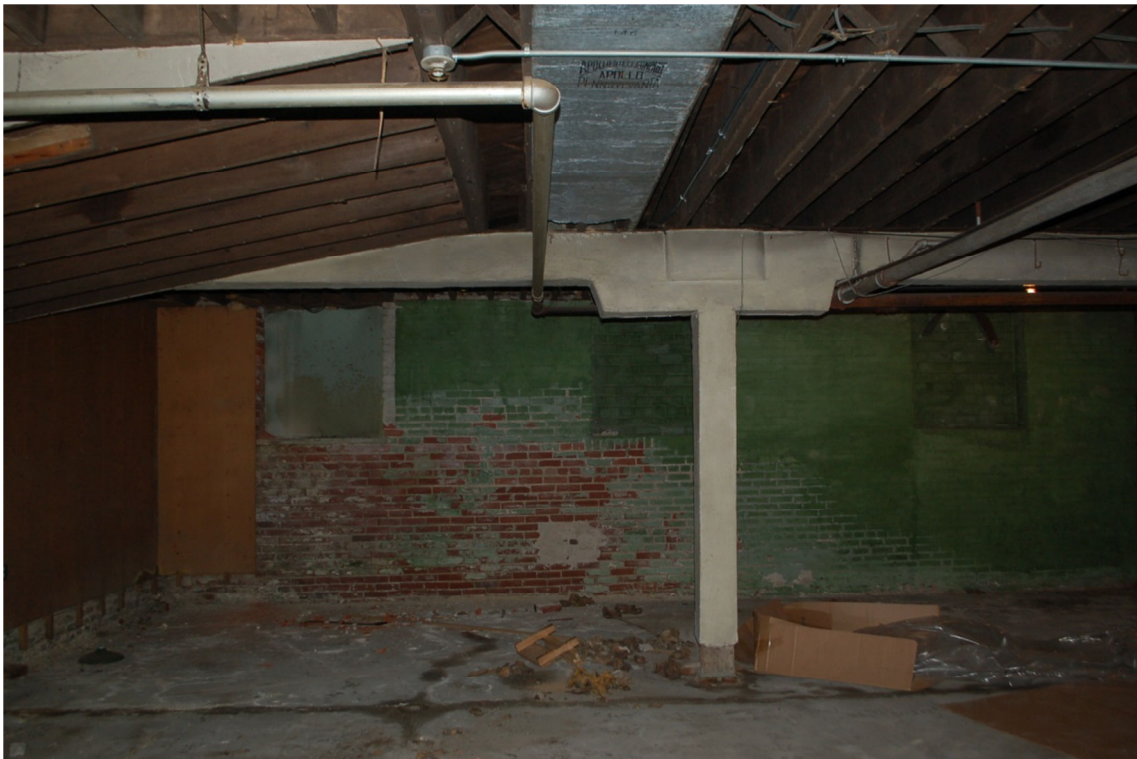
Plate H-16. Lower level of the three-story building looking west showing the wood in the support column exposed at the base (April 2, 2015).
